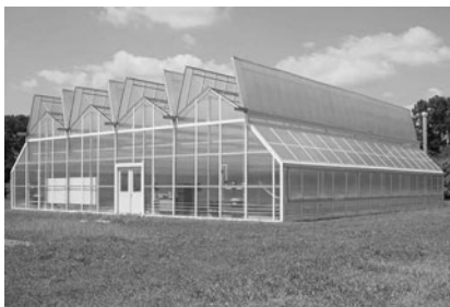
FIGURE 12–1 An open-roof greenhouse used for research at Rutgers University. (Source: Dr. AJ Both, Bioresource Engineering, Department of Plant Biology and Pathology, Rutgers University, New Brunswick, NJ 08901)
